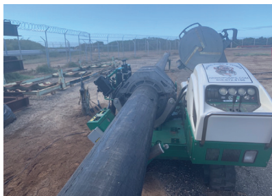
HDPE Fusion Equipment and Training
